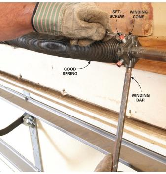
LOOSEN THE UNBROKEN SPRING Shove a winding bar into a bottom hole of the winding cone of the good spring. Hold the bar in place while you loosen the two setscrews. Hang on tight; the spring will push with powerful torque as the screws release.
