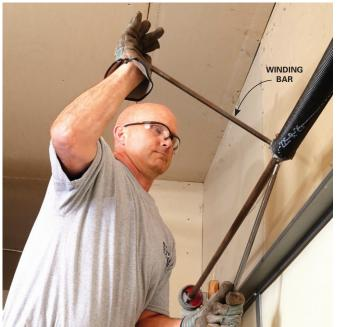
Slide a winding bar into the cone and wind toward the ceiling. Turn the spring a quarter turn at a time, leapfrogging the winding bars as you go. Follow the spring supplier's recommendations for the total number of turns. If you didn't get a recommendation, perform 30 quarter turns for a 7-ft.-tall door and 36 quarter turns for an 8-ft.-tall door.
