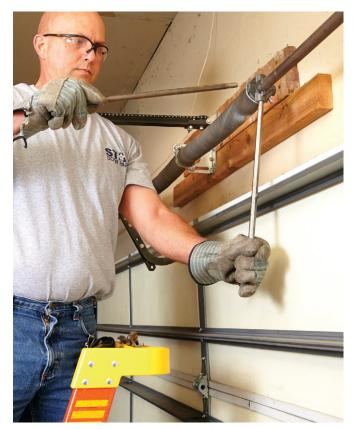
**UNWIND THE UNBROKEN SPRING** Insert the second winding bar into the hole at the 9:00 position. Remove the bottom bar and unwind the spring a quarter turn at a time, leapfrogging the winding bars with each turn.
