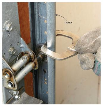
**LOCK DOWN THE DOOR** Clamp a locking pliers or a C-clamp to the track just above one of the rollers. This will prevent the door from shooting up and breaking your nose when you wind the new springs. Also yank the cord and unplug the garage door opener.
